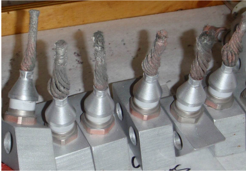
Figure 5: Wire Tied around Ends of Flexible Connectors
