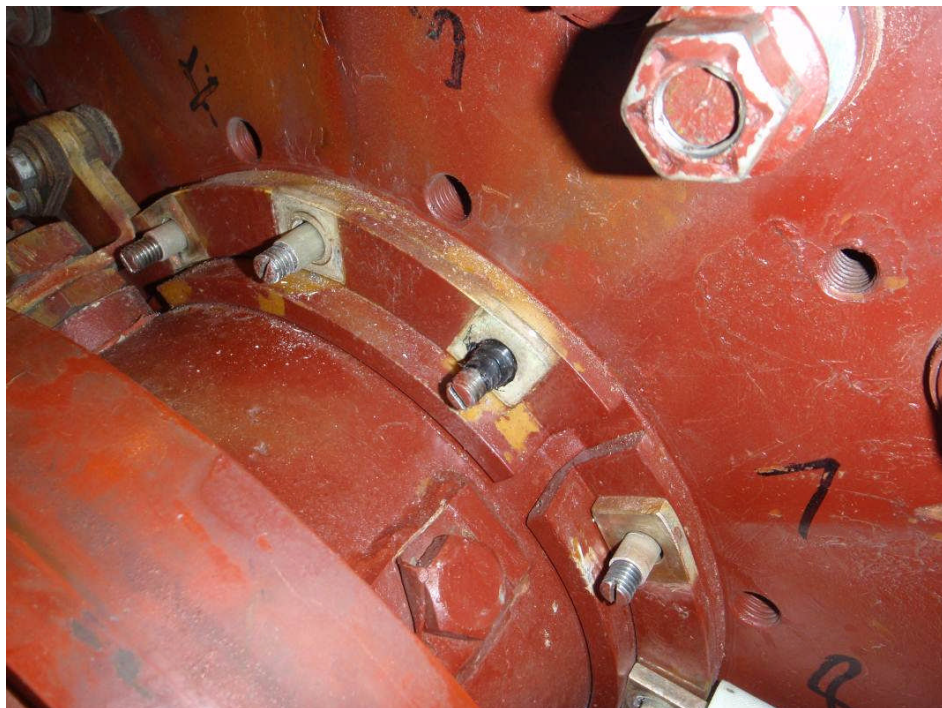
Figure 2: Missing Insulating Bushing; Replaced with Electrical Tape
